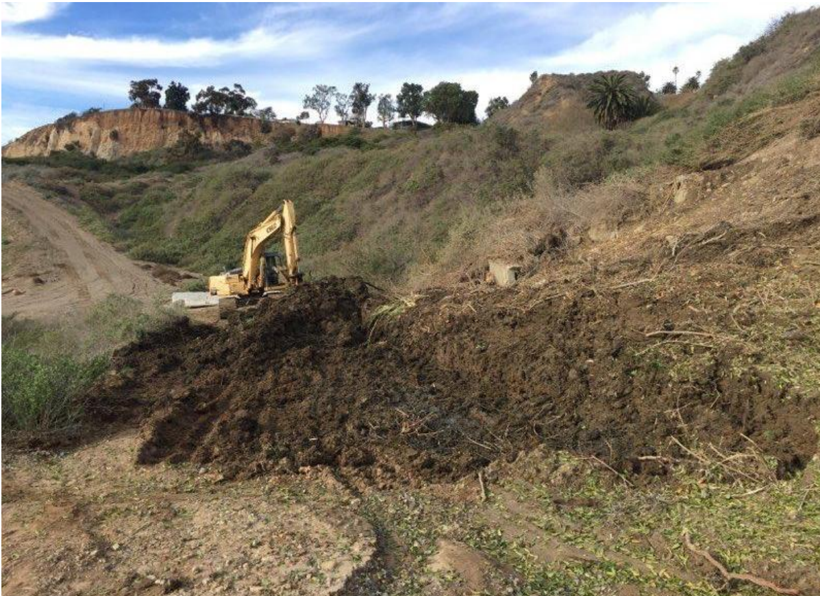
Photo 6: The Contractor excavated mud and debris, and placed geotextile on the roadway to allow safe passage from the project stockpile into the canyon and continue construction
