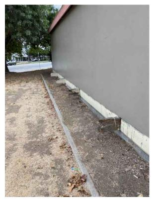
Photo 12: Exterior Eastern Portion of Building w/ Rotten Wooden Beams
