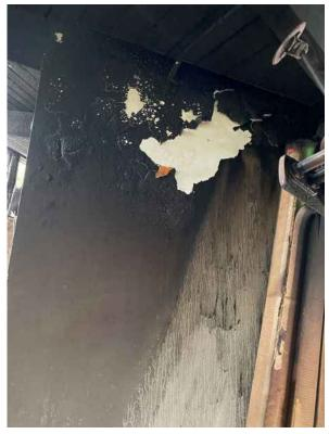
Photo 42: Coating Spalling due to Fire
