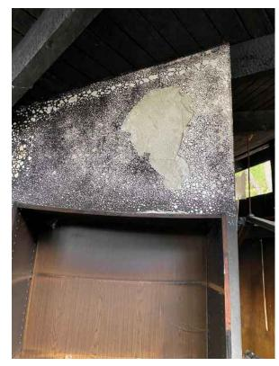
Photo 40: Coating Spalling due to Fire
