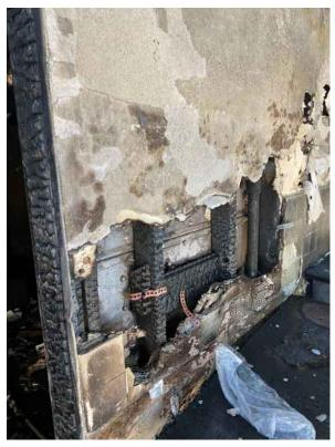
Photo 32: Damaged Portion of Bearing / Shear Wall
