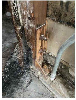
Photo 37: Typical Hold-down Seismic Connection
