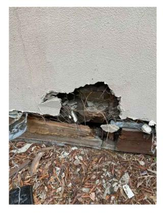
Photo 4: Existing Hole at Bottom of Building.
