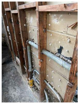
Photo 35: Exposed Portion of Wall w/ Termite Damage
