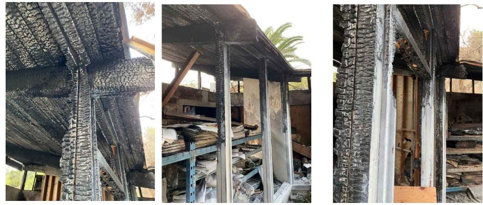
Photo 28: Interior Column and Beam w/ Size Reduction
