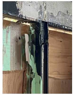
Photo 43: Cracked Interior Column due to Fire
