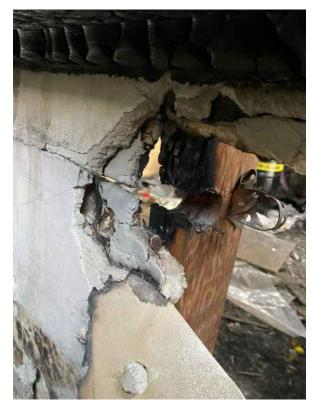
Photo 34: Burned Post of Shear Wall
