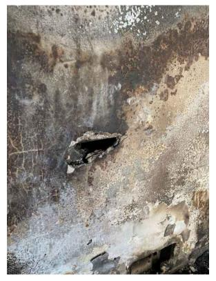
Photo 33: Burned Gypsum Board on Wall
