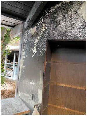
Photo 41: Coating Spalling due to Fire
