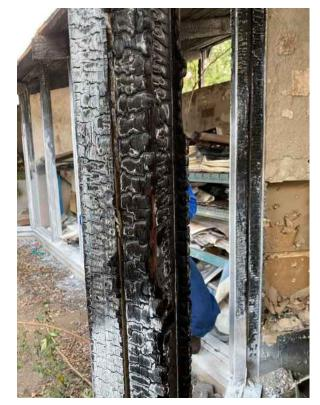
Photo 27: Burned Interior Columns at Western Side
