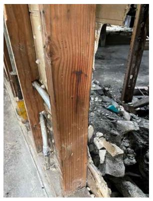
Photo 36: Typical Interior Bearing / Shear Wall
