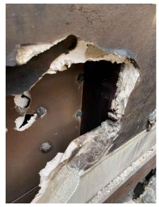
Photo 46: Burned Interior Wall Post
