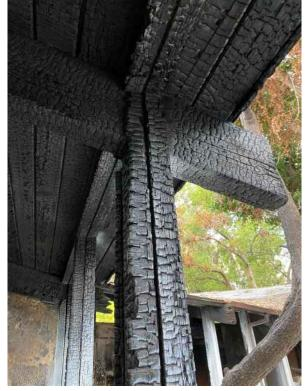
Photo 23: Burned Interior Column
