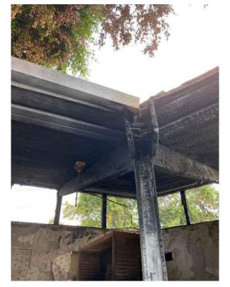
Photo 22: Burned Roof and Beams
