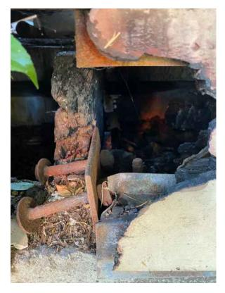
Photo 14: Burned Wood Joist for **Raised Floor**
