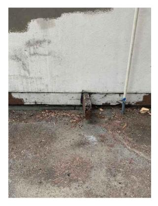
Photo 3: Rotting Wood Beam of Raised Floor On Western Portion of Building
