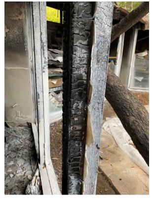
Photo 25: Burned Interior Columns at Western Side
