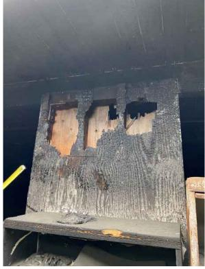
Photo 44: Heavily Burned Interior Support Wall
