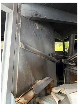
Photo 38: Undamaged Bearing / Shear Wall
