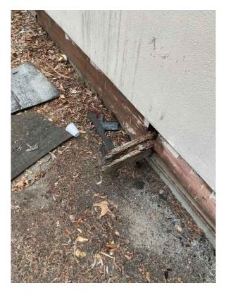
Photo 6: Rotting Wood Beams for Raise Floor
