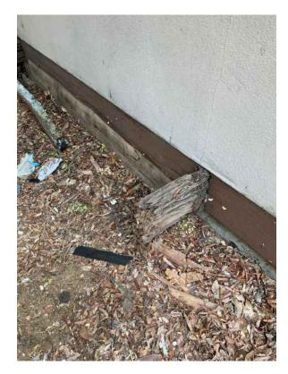
Photo 5: Rotting Wood Beams for Raise Floor
