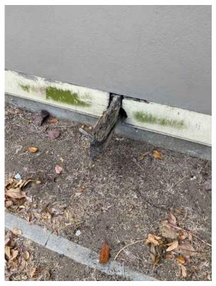
Photo 10: Rotten Wood Beam for Raised Floor
