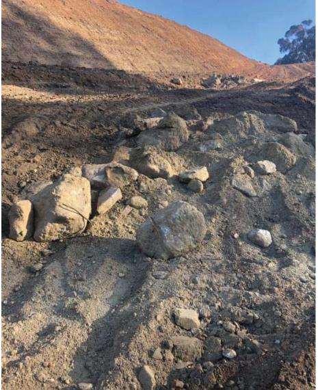
Debris such as large pieces of concrete and boulders are being found at design elevations and determined to be unsuitable for bottoms of excavation and therefore need to be removed. This is material that was used as part of a previous engineered fill constructed during the late 80s and early 90s for projects not managed by BOE.
