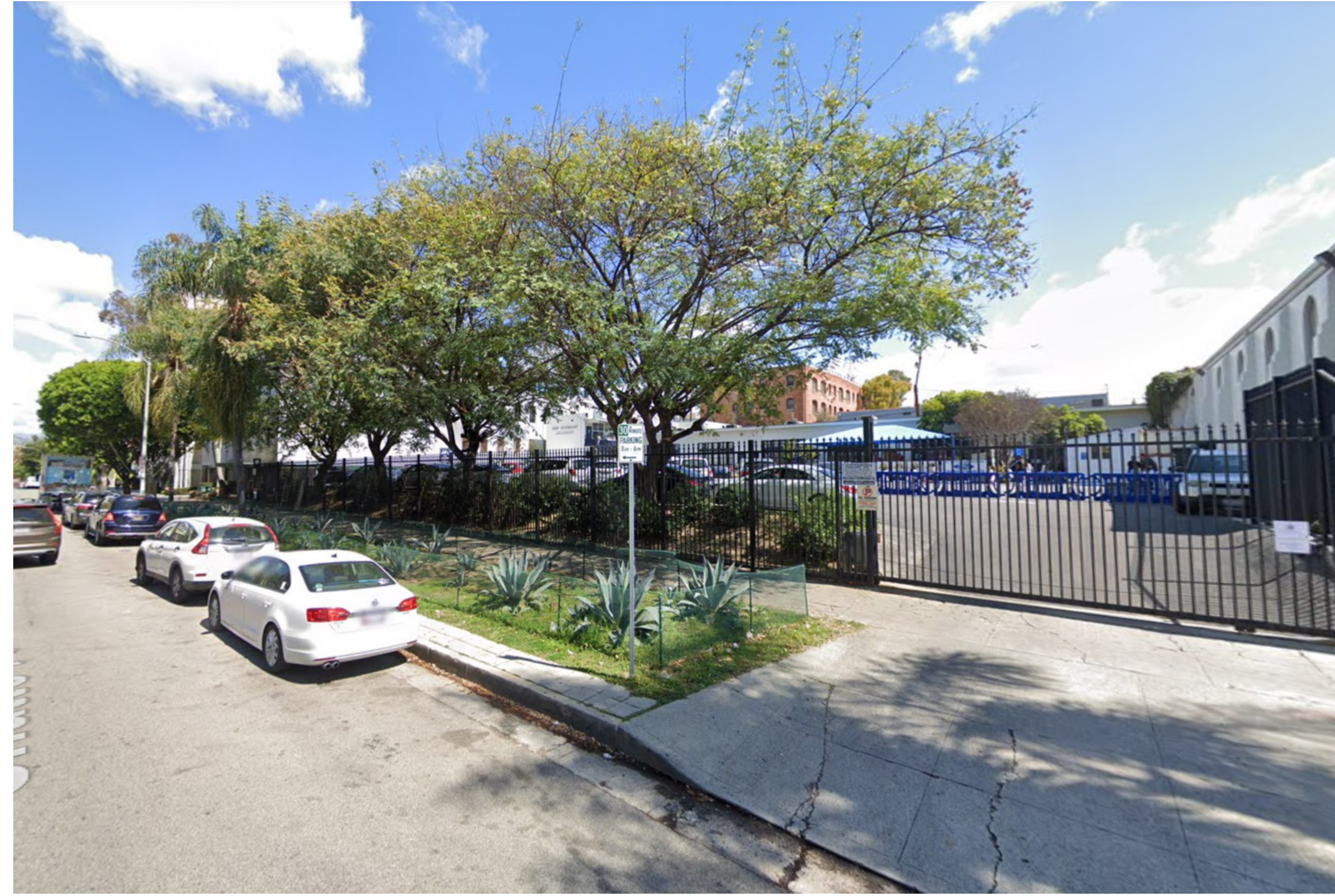
1. VIEW FROM SHATTO PL LOOKING NORTHEAST
