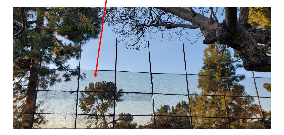
Panels with no netting leave fence at 18 ft, allowing balls to pass undeflected onto Lorenzo
