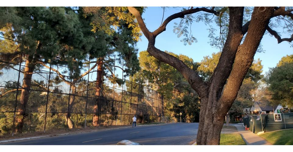
Last 4 horizontal sections of fence also only 18 ft high. Fence transitions from 18 ft to 6 ft at west end of protective fence, across from 10434 Lorenzo
