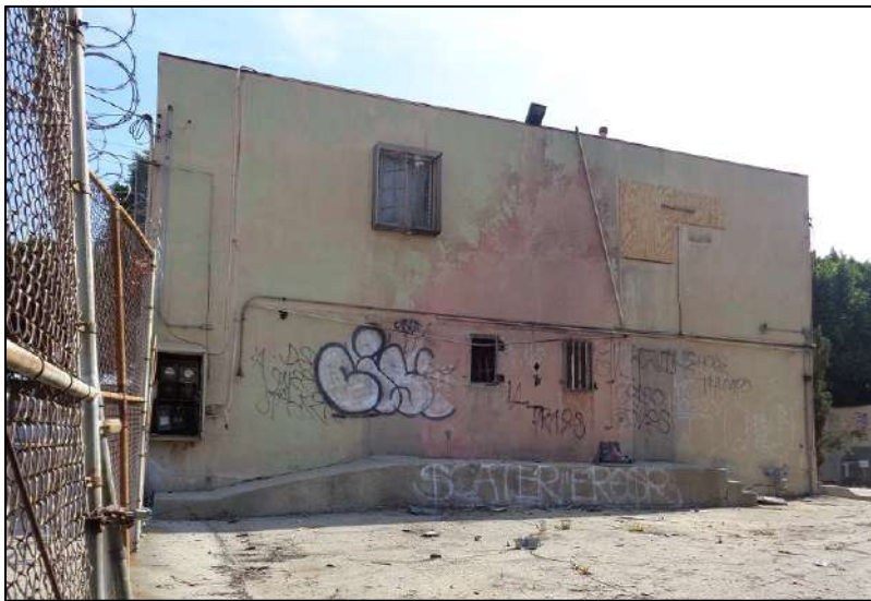
Figure 6: Rear elevation, camera facing northeast. ICF, 2018.
