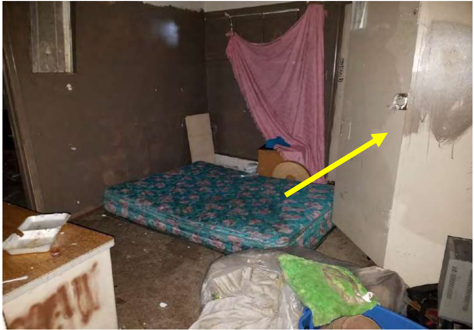
Photograph 9: Building 1: view of lead containing door.
