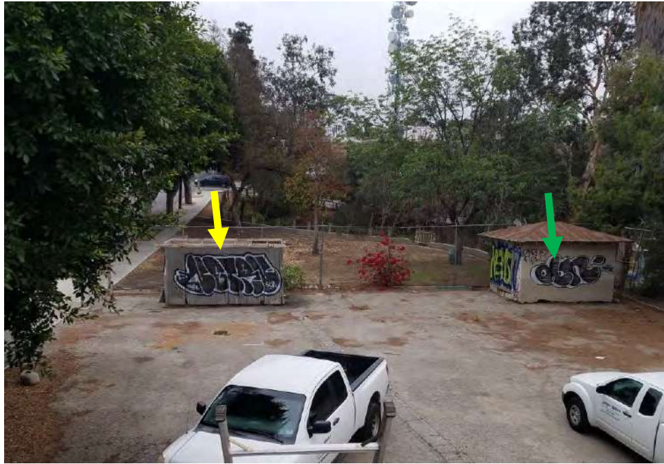
Photograph 13: General view of shed 1 (green) and shed 2 (yellow).
