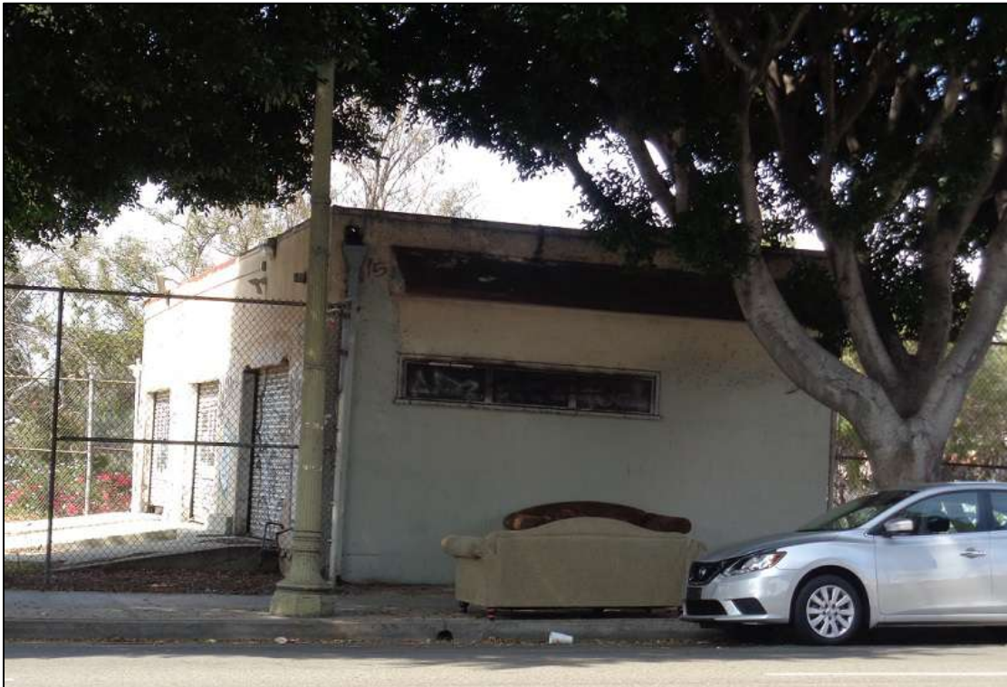
Figure 1: Primary and East Elevations, camera facing west. ICF, 2018.
