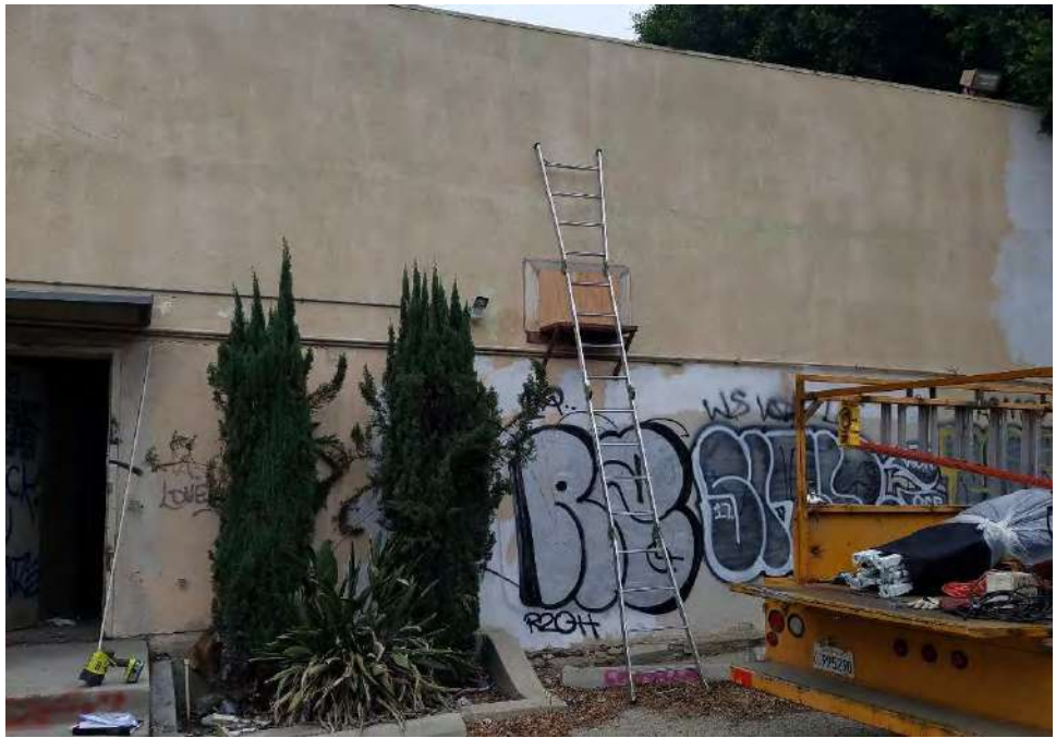
Photograph 3: Building 1: view of asbestos-containing exterior stucco.
