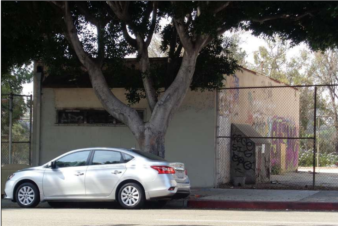
Figure 1: Primary and west elevations, camera facing south. ICF, 2018.
