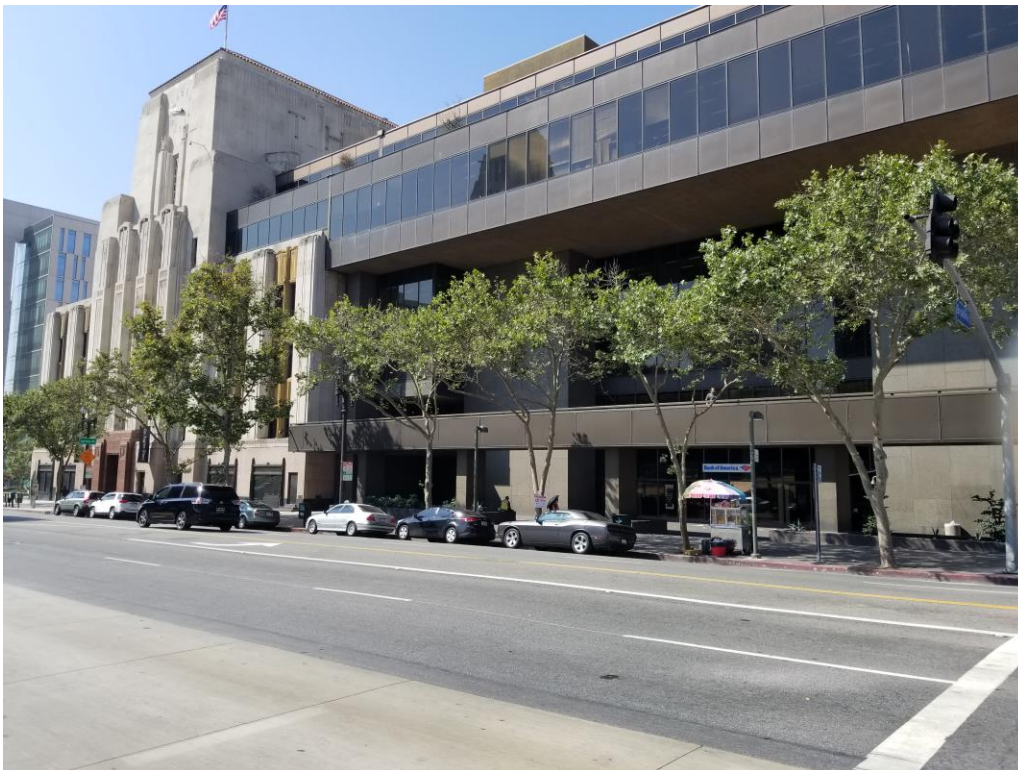
Photograph 1. Los Angeles Times Building, 202 West First Street, camera facing southeast, June 25, 2018.
