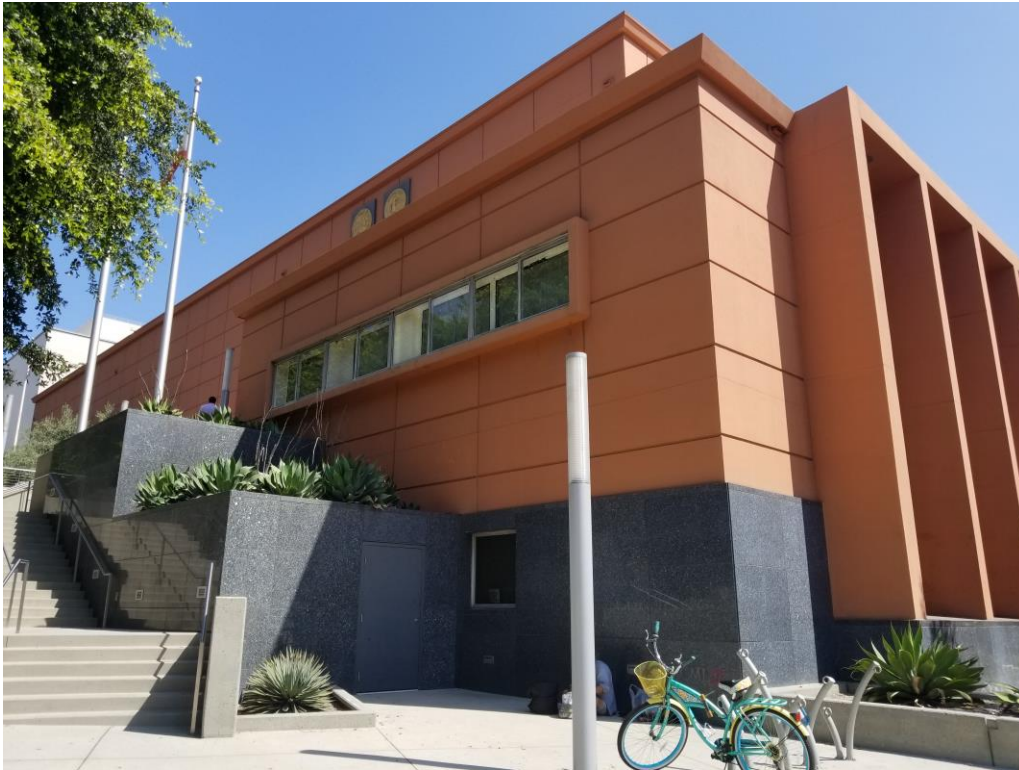
Photograph 1. Los Angeles Library, 301 West First Street, camera facing north, June 25, 2018.
