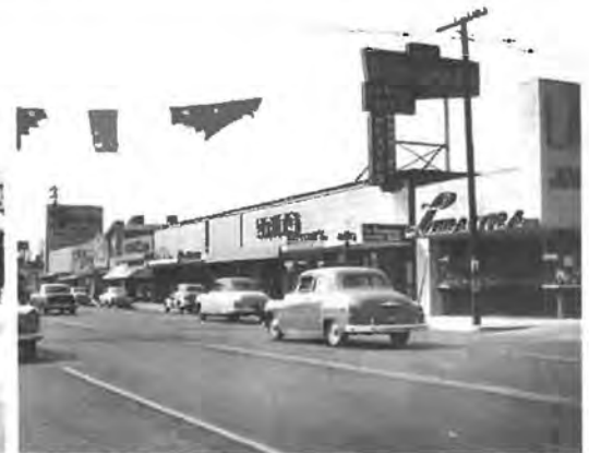
1938 LOOKING TOWARDS CANBY AVE.
