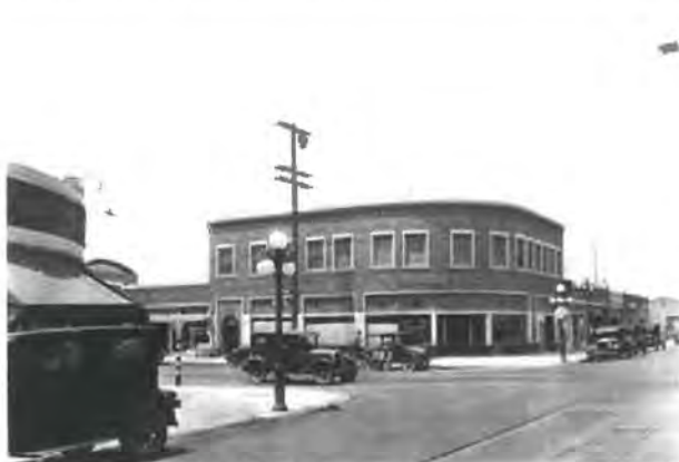
CORNER OF RESEDA BLVD.
