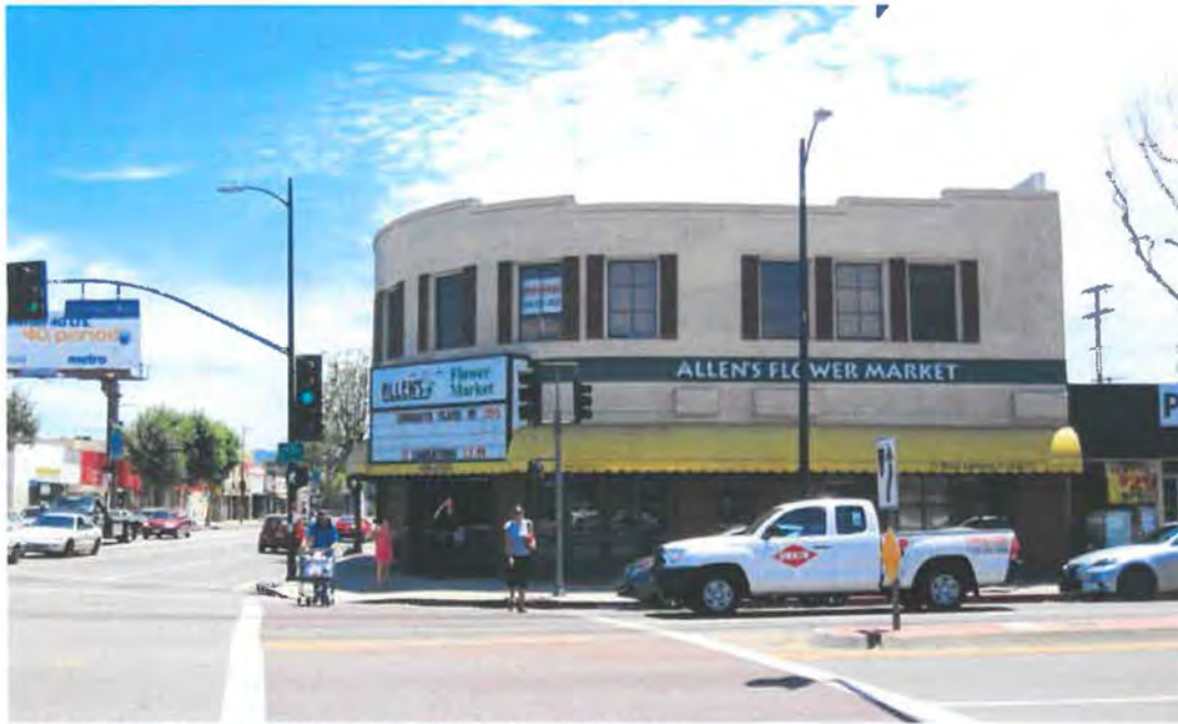
LOOKING SOUTH DOWN RESEDA BOULEVARD FROM SHERMAN WAY
