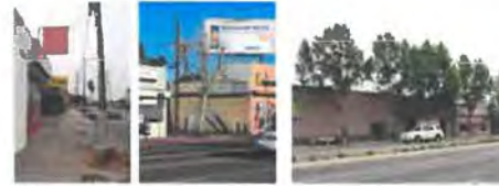
Missing and damaged trees Continuous canopy
