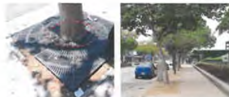
1. Enlarge opening 2. Remove grate/enlarge well
