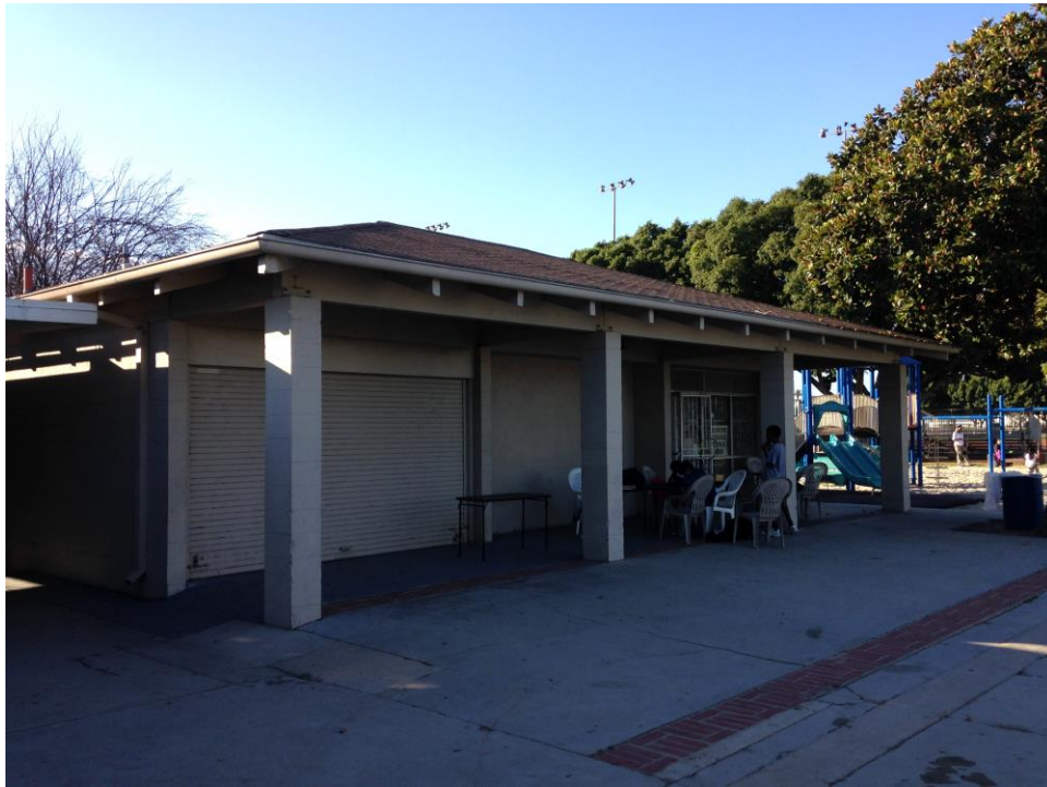
Plate 8. Tennis Shop, view facing northeast
