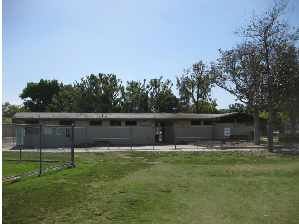
Plate 9. Restroom Facility, north side, view facing south
