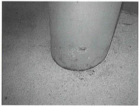
(Photo #3) Typical sand blasted base of steel column pipe.
