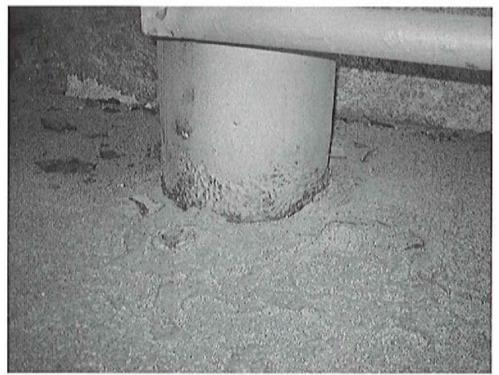
(Photo #4) Slightly damaged steel pipe due to rust.
