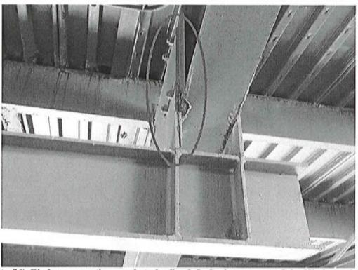
(Photo #6) Girder connection needs to be fixed. Left plate on top of the Wx beam below shall be remove and replace with new one, for plate thickness and weld, see photo #7. Plate on right side is in good condition, however needs some maintenance.
