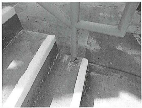
(Photo #10) Guardrail showed rust at base, needs to be repaired to its original strength.
