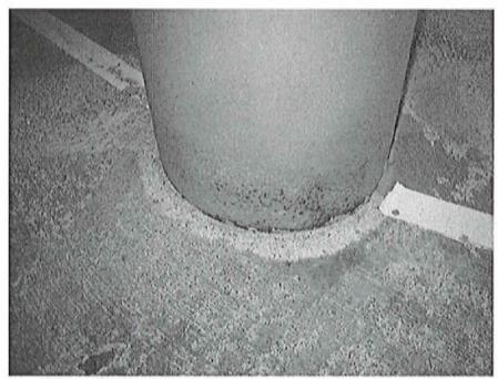
(Photo #2) Typical sand blasted base of steel column pipe.
