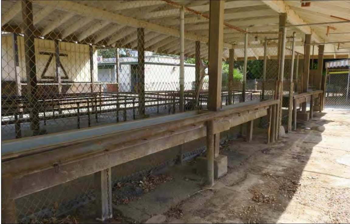
Close-up of south side of the pergola and water troughs (ARG, 2023).
