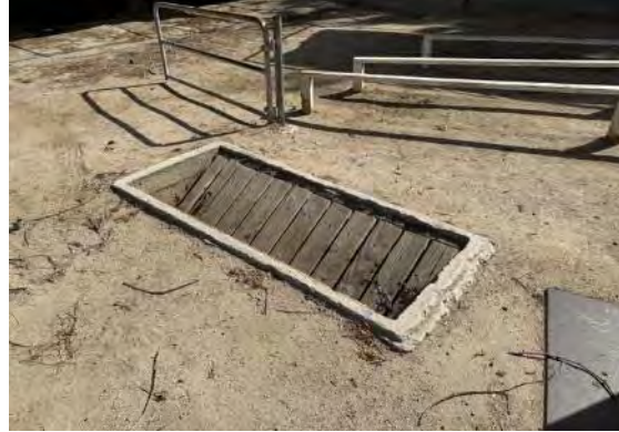
Concrete vault at north end of riding ring (ARG, 2023).
