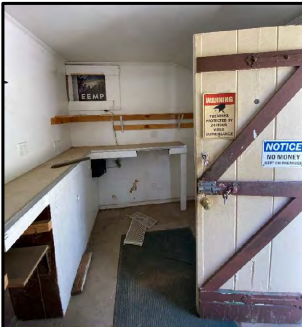
Figure 4 Interior view of the Ticket Booth showing the interior finishes.
