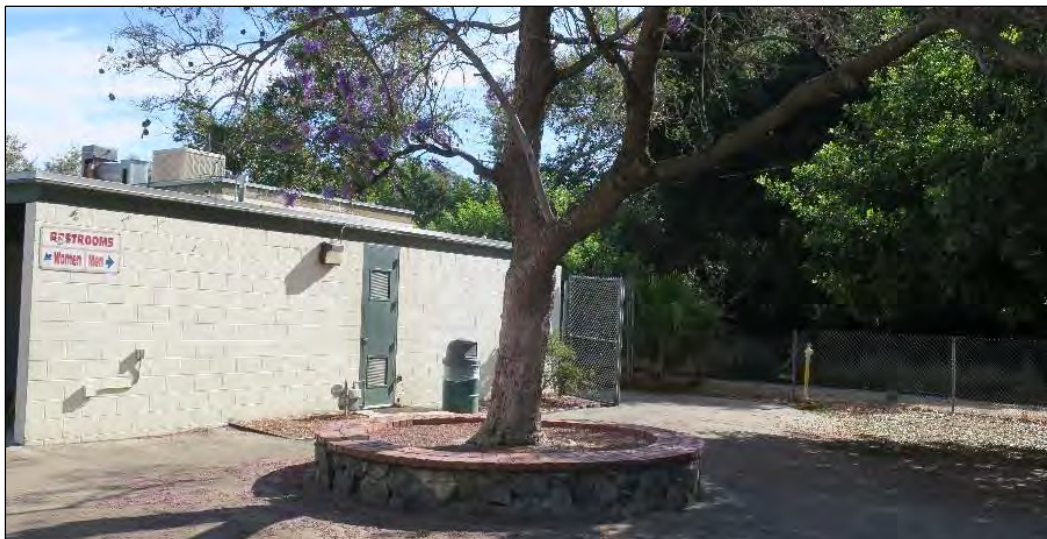
View of the masonry planter and jacaranda tree (ARG, 2023).
