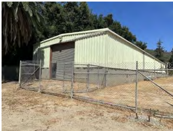
View of barn looking northwest (ARG, 2023).
