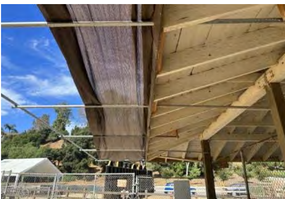
Shade structure added at south side (ARG, 2023).
