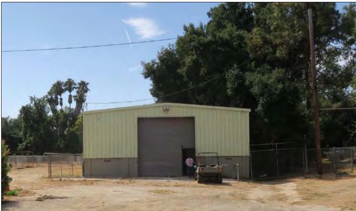
View south of the barn (ARG, 2023).
