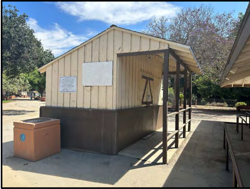
Figure 18 View of the Ticket Booth.
