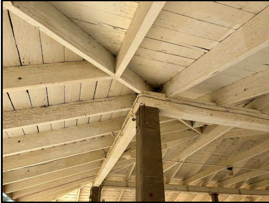
Figure 14 View of the cantilevered roof rafter framing, beams and columns.
