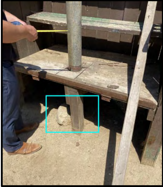
Figure 32 View of the light post foundation.
