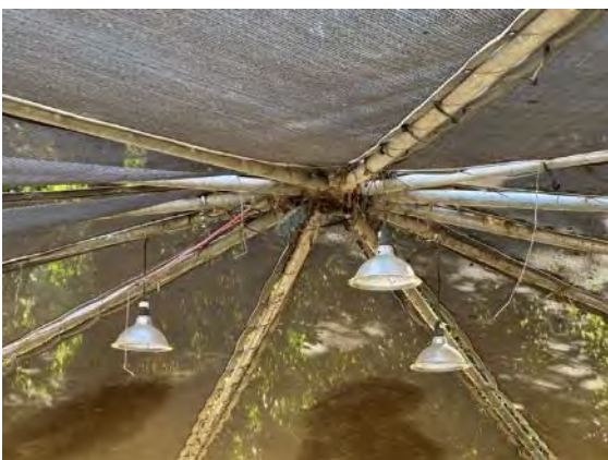
Detail at top of conical roof pipe framing and lights (ARG, 2023).
