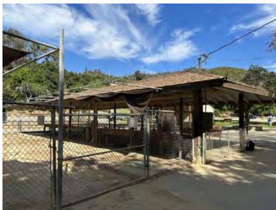
View looking northwest showing pergola and pony trough area (ARG, 2023).
