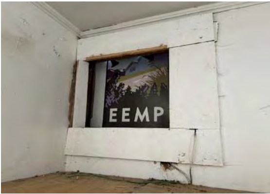
Detail at west wall A/C opening (ARG, 2023).
