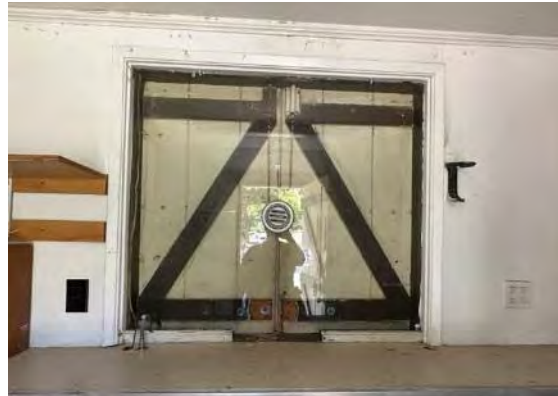
View of ticket window interior acrylic panel (ARG, 2023).
