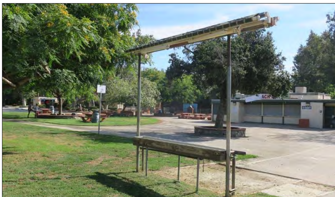
View of the freestanding shade structure (ARG, 2023).
