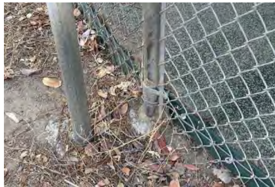
Detail at base; note pipe framing set in cement and raised interior floor (ARG, 2023).
