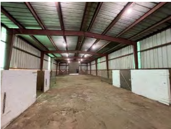
Interior view of barn looking south (ARG, 2023).
