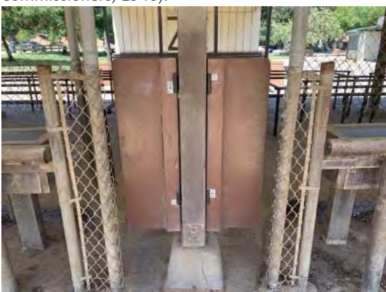
View of central pass-through with double-acting panels (ARG, 2023).
