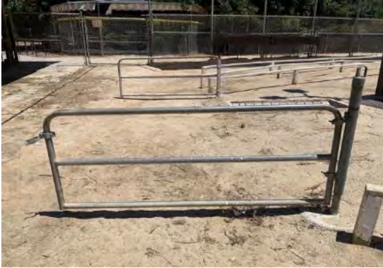
Metal gates at north end of riding ring (ARG, 2023).
