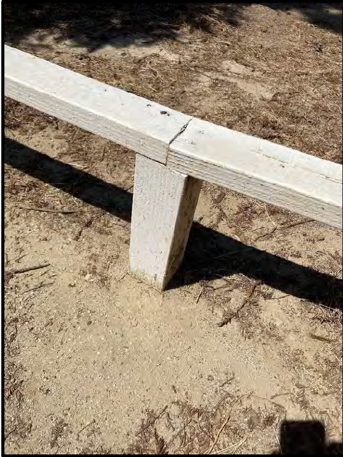
Figure 26 Close up of an Internal Guide Rail post and rail.
