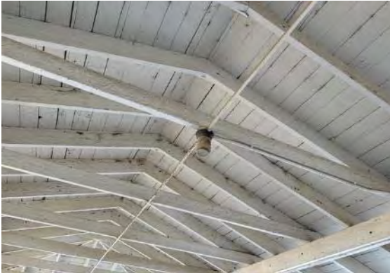
View of pergola ceiling; note light fixture and exposed conduit (ARG, 2023).
