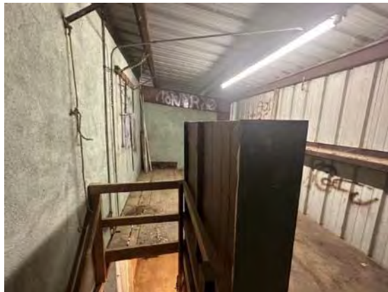
View of loft looking south (ARG, 2023).
