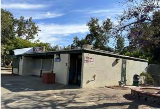
View of snack stand looking northeast (ARG, 2023).
