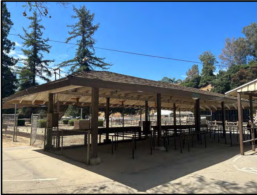
Figure 7 View of the Pergola.
