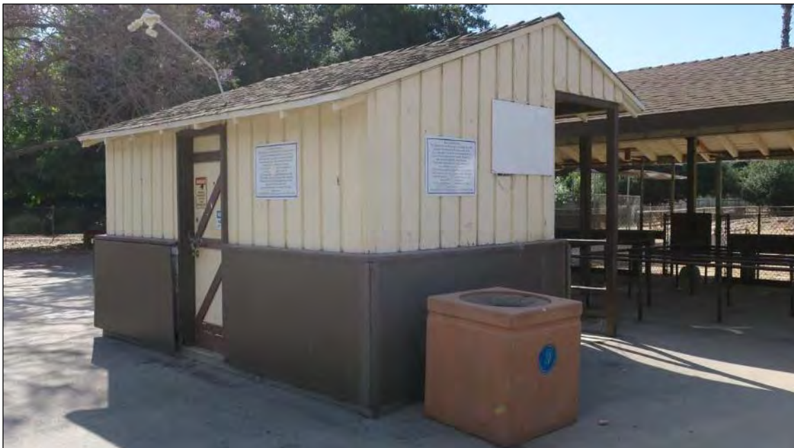
View southeast of the ticket booth (ARG, 2023).
