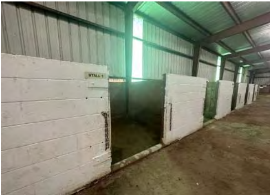
View of stalls at east side (ARG, 2023).
