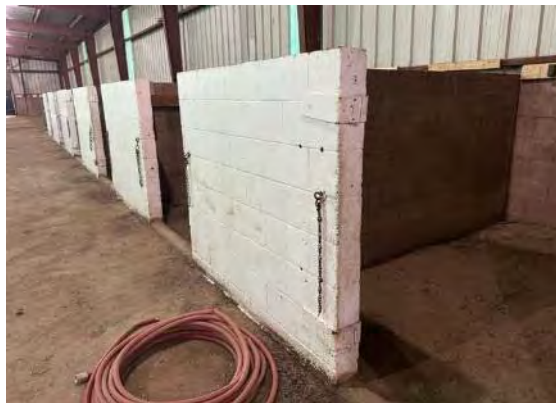
View of stalls at west side (ARG, 2023).
