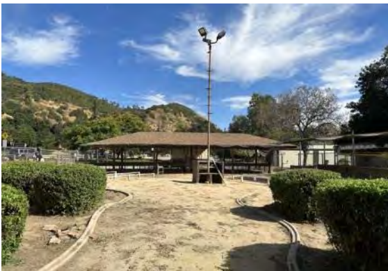
View of light post, landscaped areas, and precast concrete curbs (ARG, 2023).
