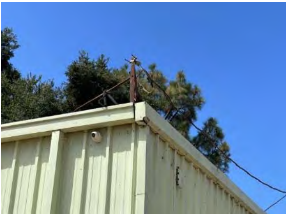
Detail at upper northeast corner/roof (ARG, 2023).
