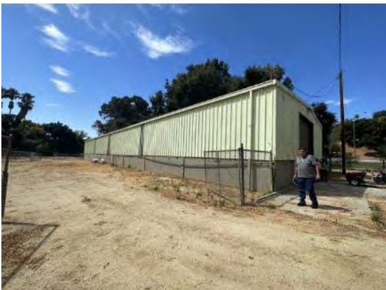
View of barn looking southwest (ARG, 2023).
