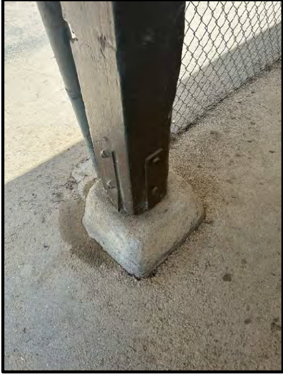
Figure 10 View of the top of the foundation.
