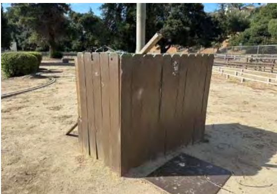
View of employee stand looking southwest; note soil collected at base (ARG, 2023).
