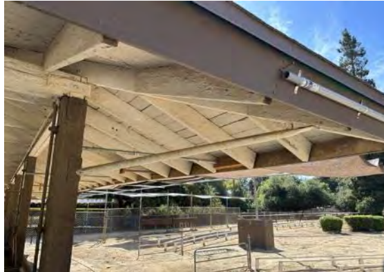
Detail at southwest corner of roof; note additional brace at overhang (ARG, 2023).
