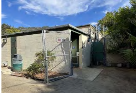
View looking northwest (ARG, 2023).
