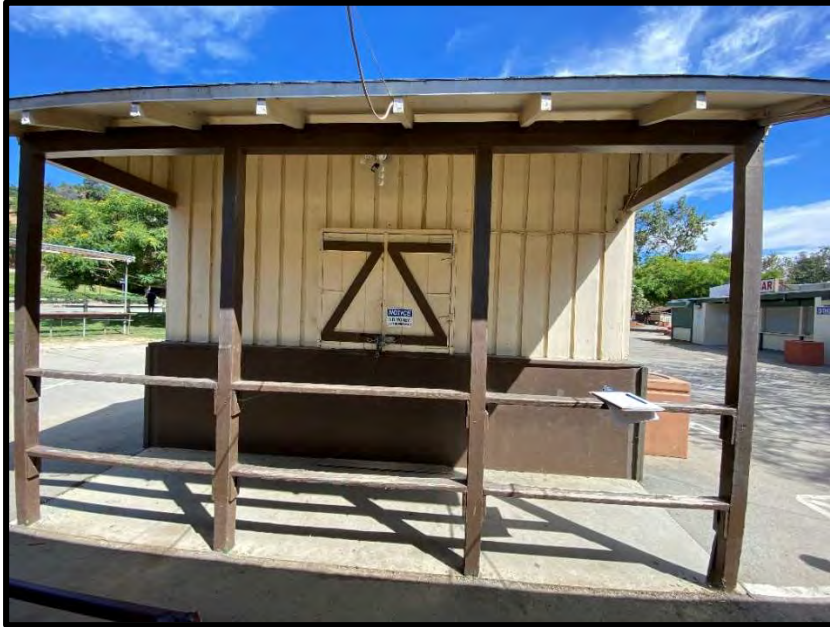
Figure 3 Exterior view of the Ticket Booth showing the exterior finishes.
