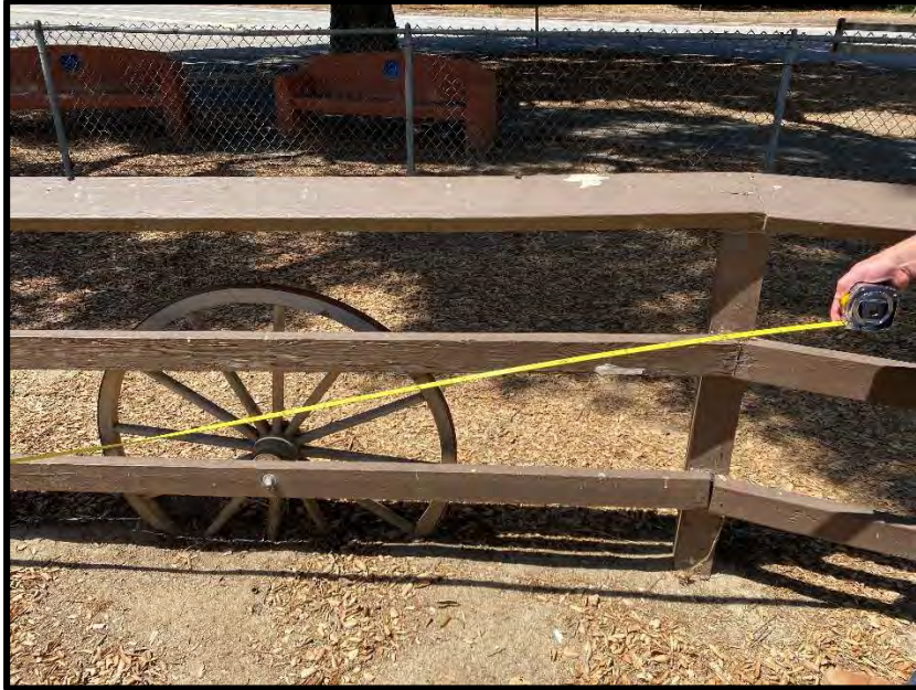
Figure 30 Close up of the Buggy Ride Guide Rail post and rail.
