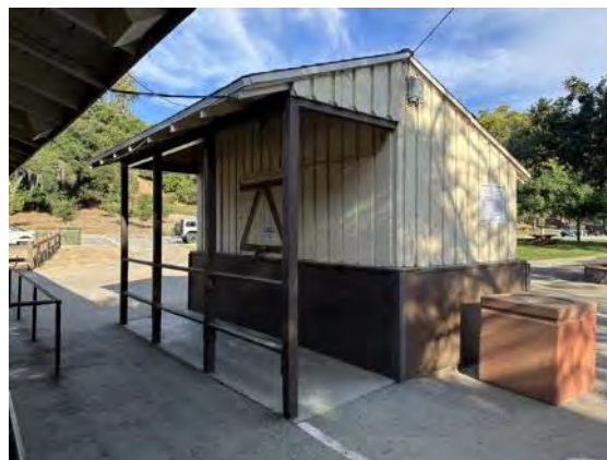
View looking northwest; note covered porch and ticket window (ARG, 2023).
