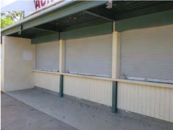
View of snack bar order/pick-up windows with roll-up shutters (ARG, 2023).
